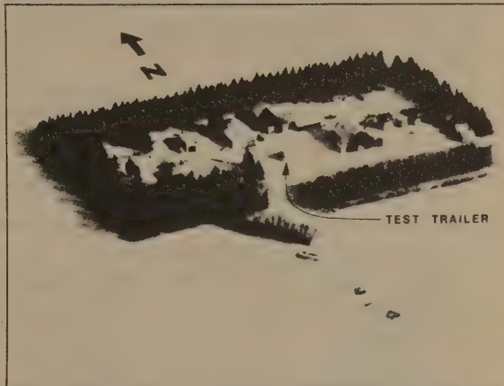
Unsheltered test trailer site (above); in the sheltered site (below), the trailer used 22.3 percent less electricity.
